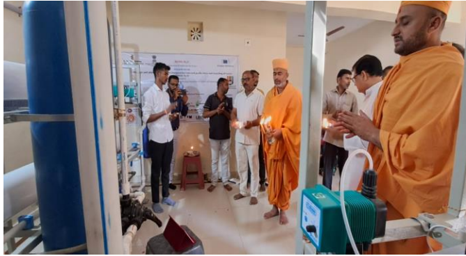
Inauguration of Batch RO- FO unit
