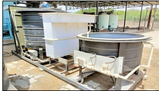
Pilot scale electrocoagulation unit is established to remove suspended, emulsified or dissolved contaminants from wastewater using direct electric current.
